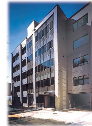
総合研究棟 H棟 H Hall (Intergrated Projects Research Center)
