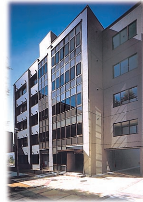
総合研究棟 H棟 H Hall (Intergrated Projects Research Center)
